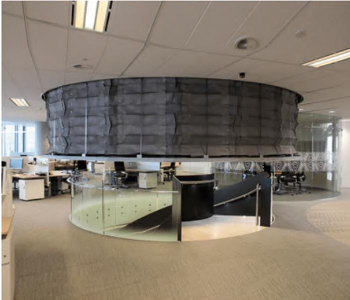
Providing and fixing of “ENVIROTECH” Automatic fire Curtain The Fire Curtain is an automatic, fire protective barrier that prevents fire and smoke from transferring from one part of a building to another. The Fire Protective Curtain is a vertical deploying opening protective, ideal to replace fire doors and protect atriums and lobbies.
