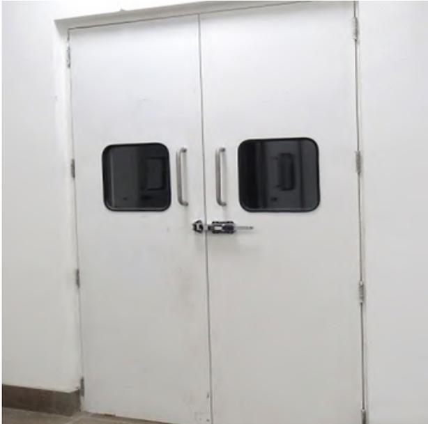
Envirotech Systems is a leading manufacturer of Metal Acoustic Doors in India. Metal Acoustic Doors are essential whenever high sound reduction performance is required between noise-sensitive areas.
