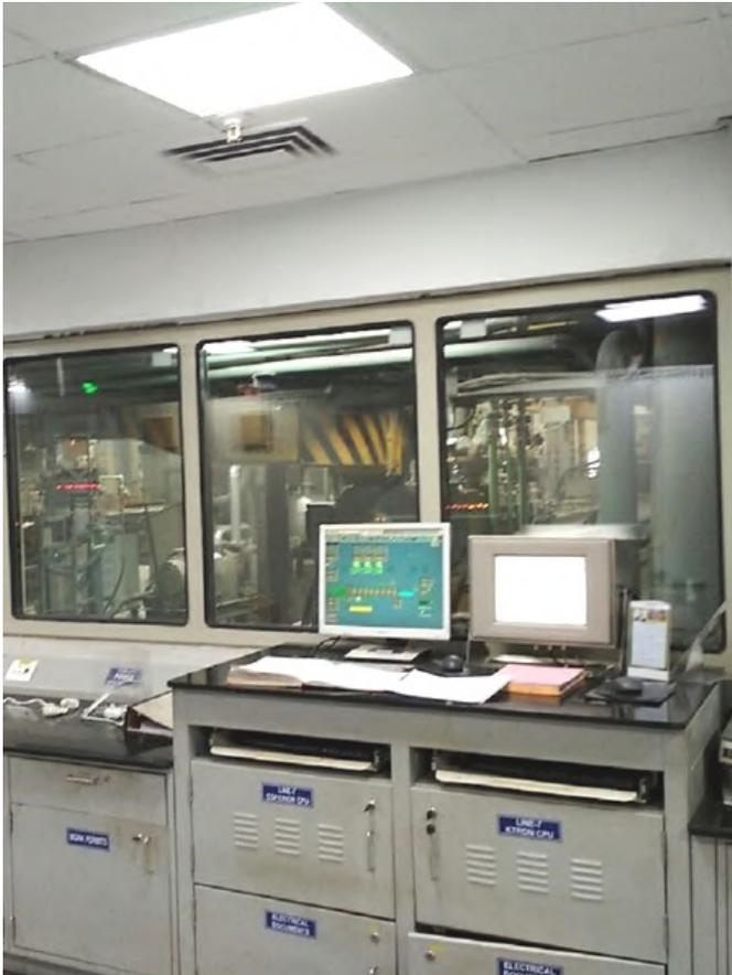
ENVIROTECH MAKE Acoustic Window that offers sound reduction up to 40dB. Acoustic window glass having 2 or 3 nos. toughened glass with argon gas filled in between that offers high sound reduction. Acoustic windows are fitted with Acoustic seals and silicon sealing for best performance.
